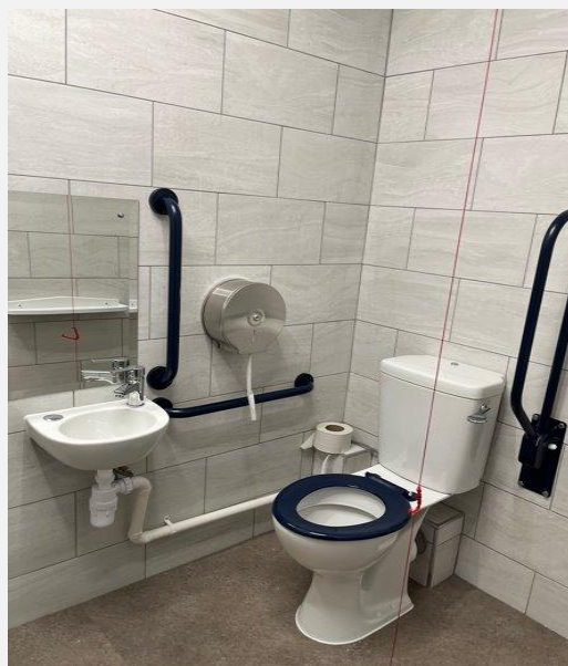
Inside layout of an accessible toilet
